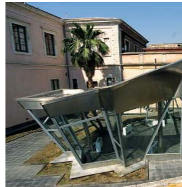
Arezzo Courthouse (2001-2007) refurbishment and extension built
